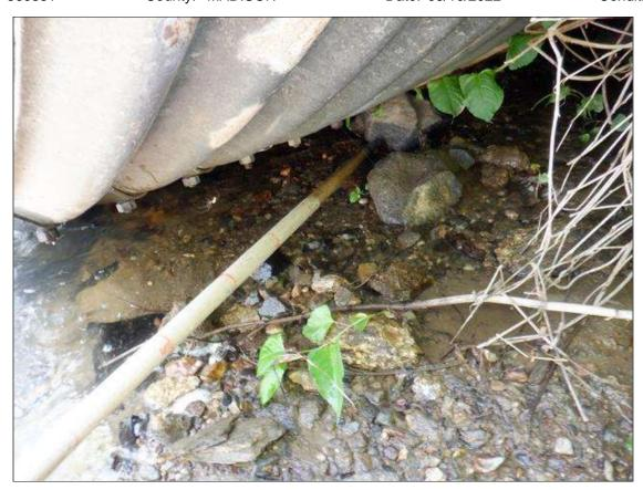
Span 3 Culvert Section 12: FULL WIDTH X 2.5' HIGH X 3' BACK SCOUR AT THE OUTLET END.
