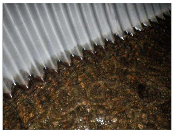
Span 2 Culvert Section 2: CORROSION WITH 0.0625" PITTING AND SCALE LOSS ALONG THE WATERLINE. BOTTOM PORTION NOT VISIBLE DUE TO ROCK AND SEDIMENT BUILDUP.
