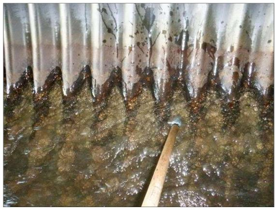
Span 3 Culvert Section 12: CORROSION WITH UP TO 0.0625" PITTING ALONG THE INVERT, UNDERNEATH THE WATER LINE.
