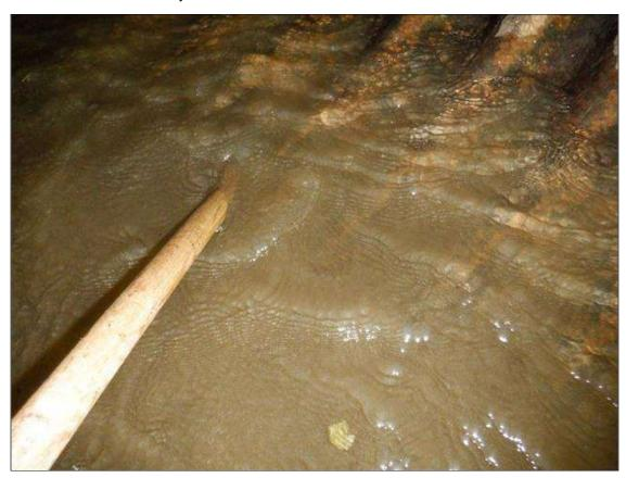
Span 1 Culvert Section 7: SEDIMENT AND ROCK HAS WASHED OUT OF THE PIPE EXPOSING THE INVERT. CORROSION WITH MULTIPLE AREAS OF COMPLETE LOSS IN THE CORRUGATIONS UP TO 5' WIDE X 3" LONG. THE STREAM IS INTRUDING UNDERNEATH THE CULVERT. (PAR)
