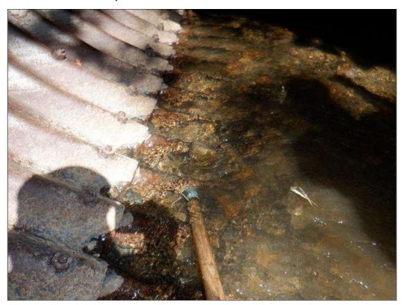
Span 1 Culvert Section 1: SEDIMENT AND ROCK HAS WASHED OUT OF THE PIPE EXPOSING THE INVERT. CORROSION WITH MULTIPLE AREAS OF COMPLETE LOSS IN THE CORRUGATIONS UP TO 5' WIDE X 3" LONG. THE STREAM IS INTRUDING UNDERNEATH THE CULVERT. (PAR)
