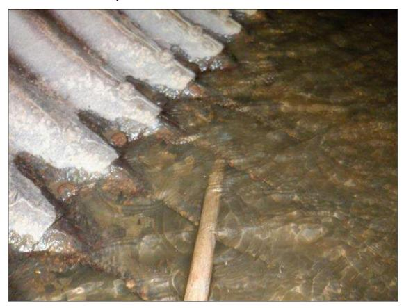
Span 1 Culvert Section 3: SEDIMENT AND ROCK HAS WASHED OUT OF THE PIPE EXPOSING THE INVERT. CORROSION WITH MULTIPLE AREAS OF COMPLETE LOSS IN THE CORRUGATIONS UP TO 5' WIDE X 3" LONG. THE STREAM IS INTRUDING UNDERNEATH THE CULVERT. (PAR)
