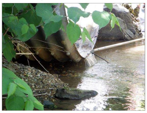
Span 1 Culvert Section 12: FULL WIDTH X 0.5' HIGH X 3' BACK SCOUR AT THE OUTLET END.
