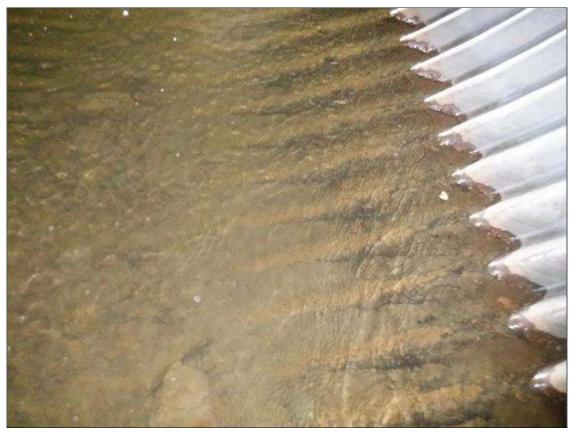
Span 2 Culvert Section 3: CORROSION WITH 0.0625" PITTING AND SCALE LOSS ALONG THE WATERLINE. BOTTOM PORTION NOT VISIBLE DUE TO ROCK AND SEDIMENT BUILDUP.
