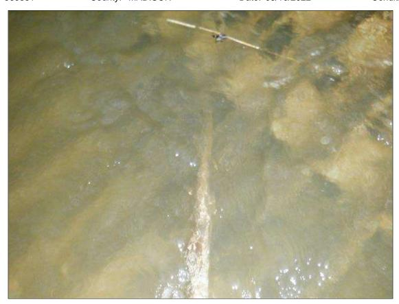
Span 3 Culvert Section 1: SEDIMENT AND ROCK WASHED OUT OF PIPE FOR 25' BEGINNING AT THE INLET. EXPOSED MULTIPLE AREAS OF COMPLETE LOSS IN THE CORRUGATIONS UP TO 5' WIDE X 6" DEEP. (PAR)
