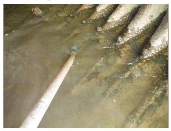
Span 1 Culvert Section 8: SEDIMENT AND ROCK HAS WASHED OUT OF THE PIPE EXPOSING THE INVERT. CORROSION WITH MULTIPLE AREAS OF COMPLETE LOSS IN THE CORRUGATIONS UP TO 5' WIDE X 3" LONG. THE STREAM IS INTRUDING UNDERNEATH THE CULVERT. (PAR)
