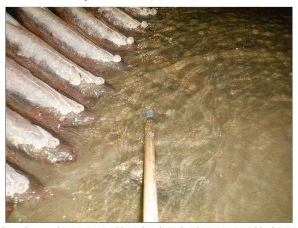
Span 1 Culvert Section 5: SEDIMENT AND ROCK HAS WASHED OUT OF THE PIPE EXPOSING THE INVERT. CORROSION WITH MULTIPLE AREAS OF COMPLETE LOSS IN THE CORRUGATIONS UP TO 5' WIDE X 3" LONG. THE STREAM IS INTRUDING UNDERNEATH THE CULVERT. (PAR)
