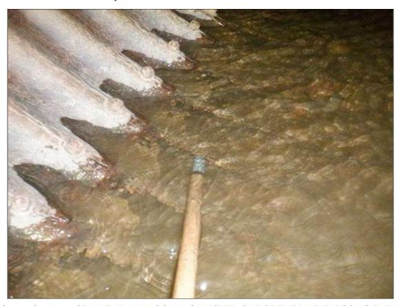
Span 1 Culvert Section 4: SEDIMENT AND ROCK HAS WASHED OUT OF THE PIPE EXPOSING THE INVERT. CORROSION WITH MULTIPLE AREAS OF COMPLETE LOSS IN THE CORRUGATIONS UP TO 5' WIDE X 3" LONG. THE STREAM IS INTRUDING UNDERNEATH THE CULVERT. (PAR)
