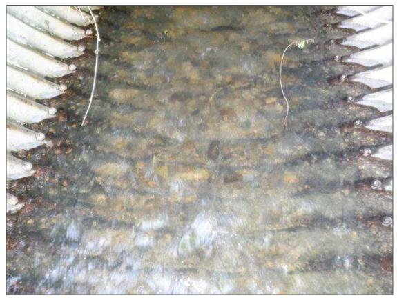
Span 2 Culvert Section 1: CORROSION WITH 0.0625" PITTING AND SCALE LOSS ALONG THE WATERLINE. BOTTOM PORTION NOT VISIBLE DUE TO ROCK AND SEDIMENT BUILDUP.
