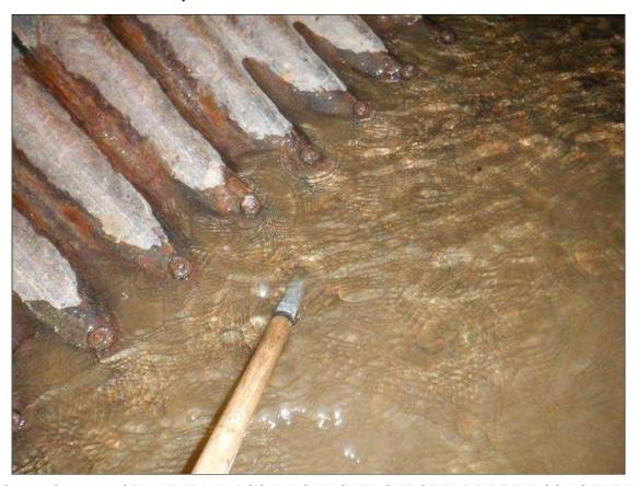
Span 1 Culvert Section 6: SEDIMENT AND ROCK HAS WASHED OUT OF THE PIPE EXPOSING THE INVERT. CORROSION WITH MULTIPLE AREAS OF COMPLETE LOSS IN THE CORRUGATIONS UP TO 5' WIDE X 3" LONG. THE STREAM IS INTRUDING UNDERNEATH THE CULVERT. (PAR)
