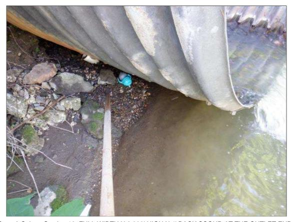
Span 2 Culvert Section 12: FULL WIDTH X 2.333' HIGH X 4' BACK SCOUR AT THE OUTLET END.
