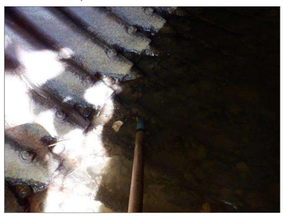
Span 1 Culvert Section 2: SEDIMENT AND ROCK HAS WASHED OUT OF THE PIPE EXPOSING THE INVERT. CORROSION WITH MULTIPLE AREAS OF COMPLETE LOSS IN THE CORRUGATIONS UP TO 5' WIDE X 3" LONG. THE STREAM IS INTRUDING UNDERNEATH THE CULVERT. (PAR)
